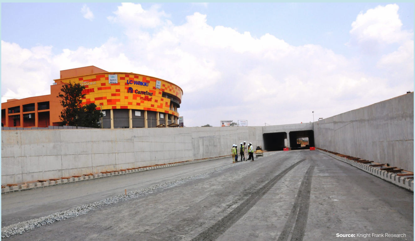
A section of the completed Kampala Flyover adjacent to the Arena Mall Nsambya
