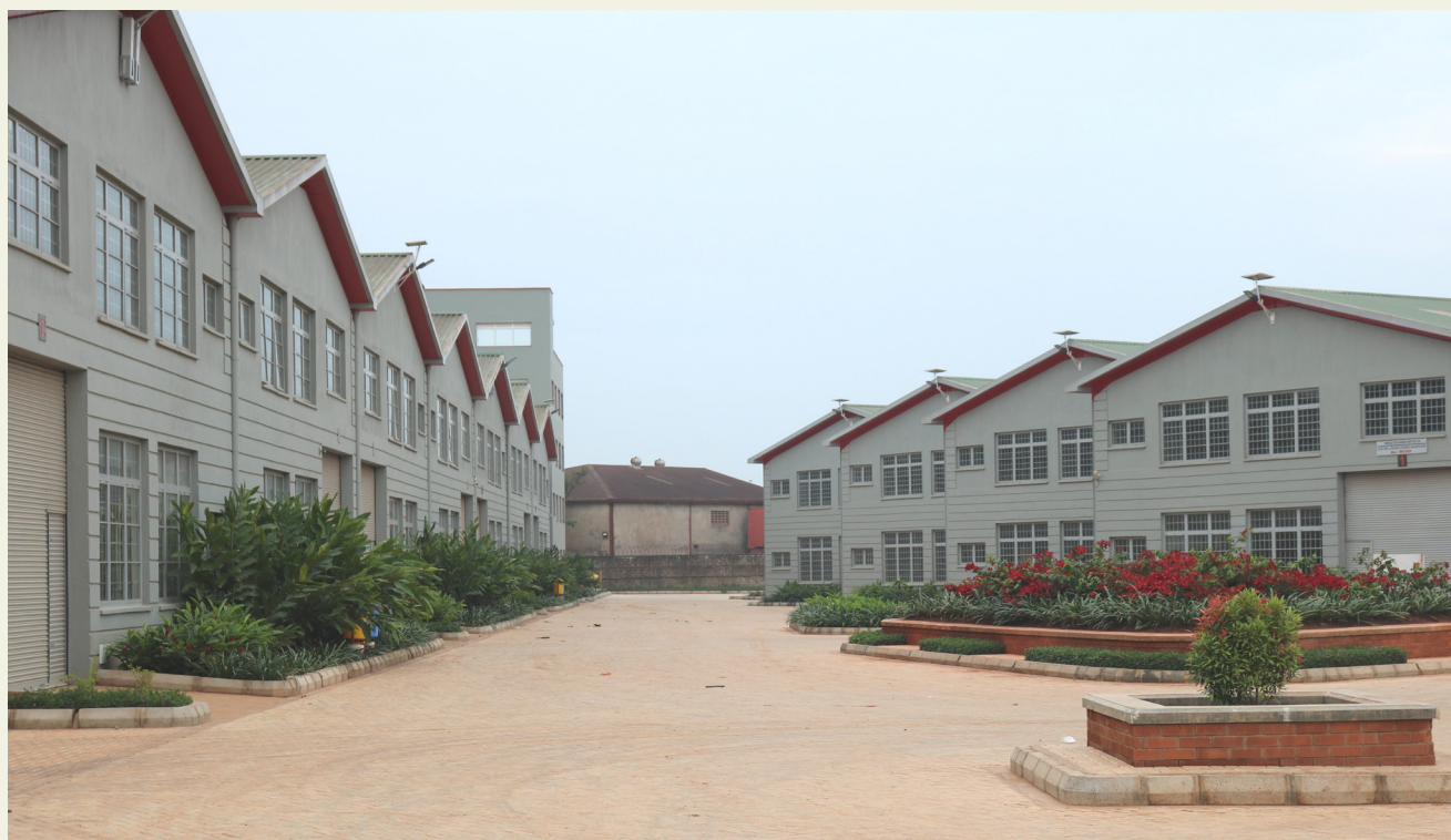
Yogi Industrial Park Nalukolongo
