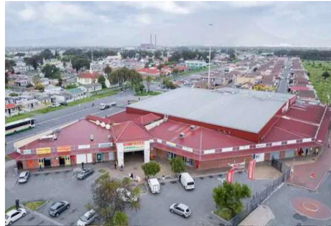
Langa Junction Brinton St, Cape Town
