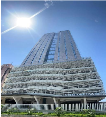
Greystone Tower, Victoria Island, Lagos
