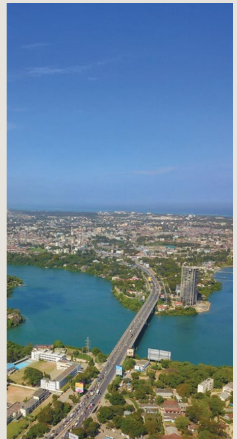
IMAGE: Mombasa Nyali Bridge
