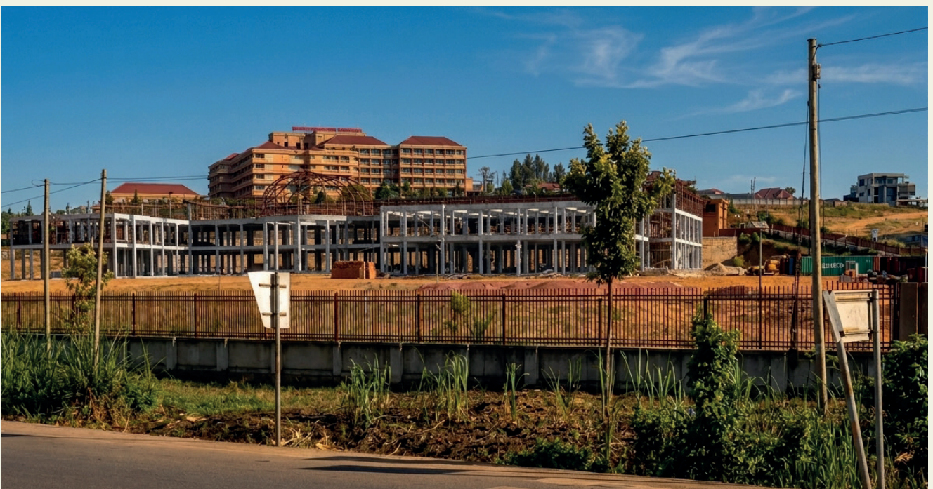
Construction progress of Mbarara Mall. Source: Knight Frank
