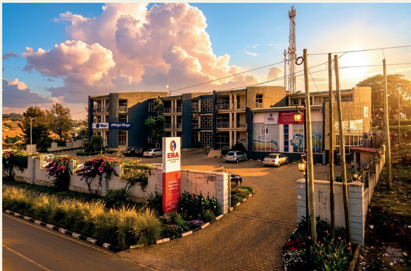
Prime Office Building in Boma
