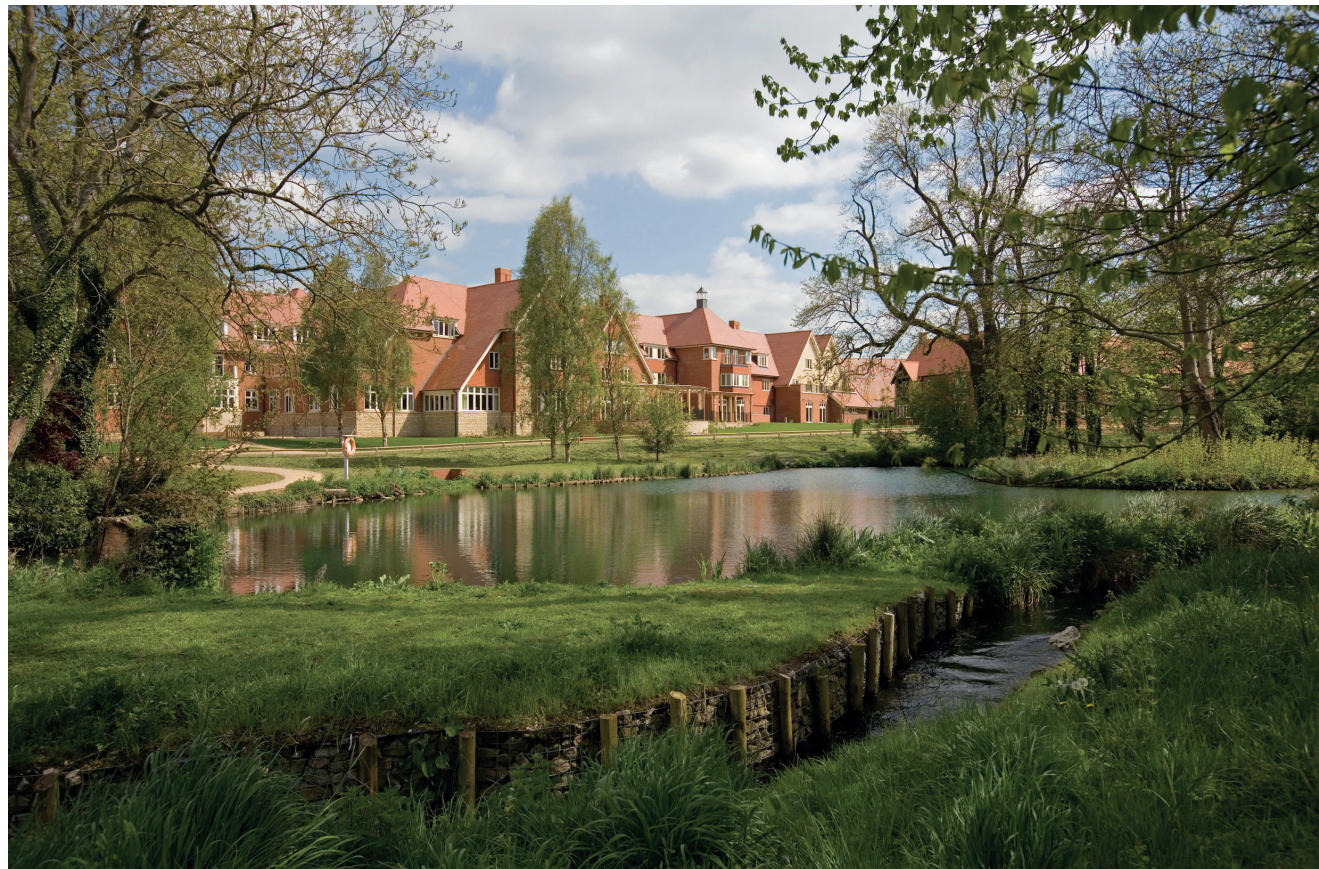
Retirement Village Letcombe Regis, Richmond Villages (part of Bupa), Castloak Development
