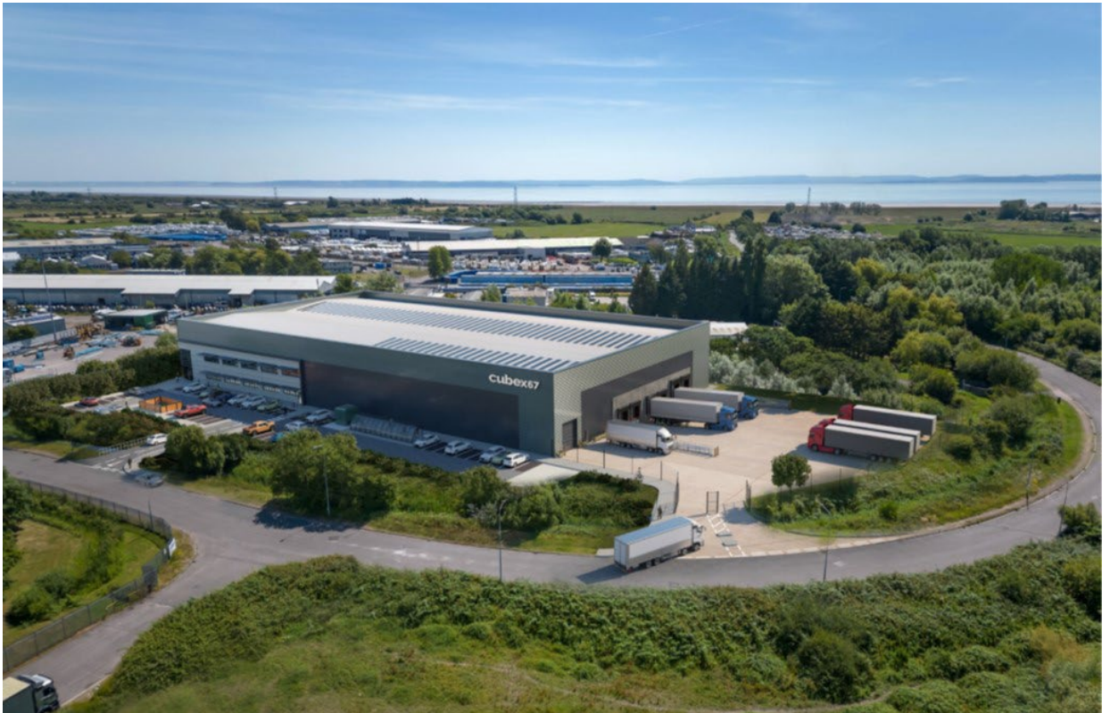
CGI image: 67,500 sq ft planned new build at Wentloog, Cardiff Development by Cubex Land
