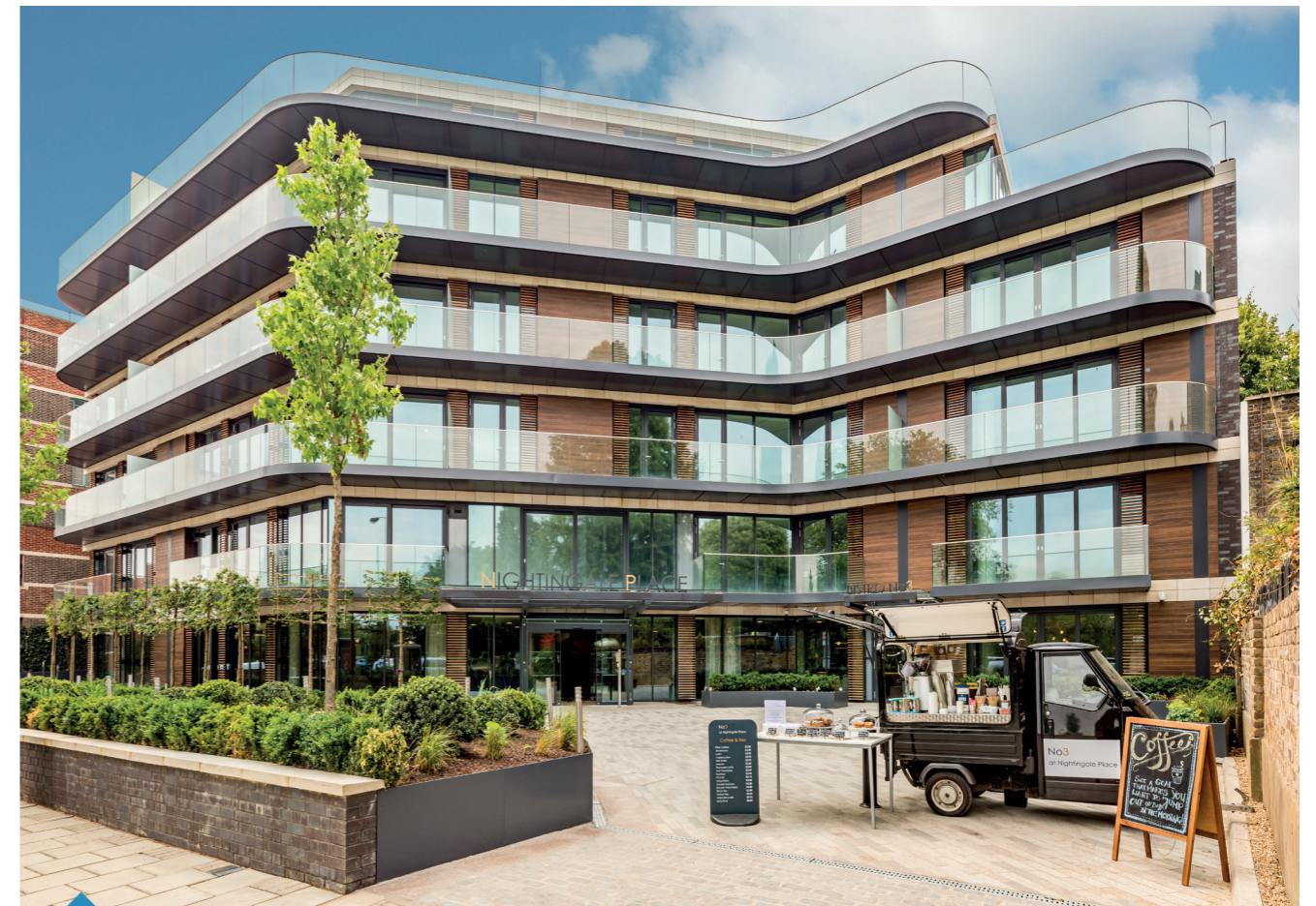
Pictured above: Audley Villages' Nightingale Place development in Clapham. In 2020, Audley Villages entered into a JV with Danish pension group PFA to form Evia Living, a new integrated retirement community platform in Denmark.
