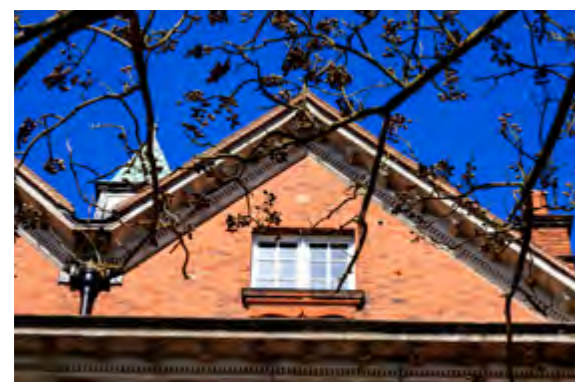
The red-bricked gable of Chapman supports a proud cornice with detail brackets from Roman cement
