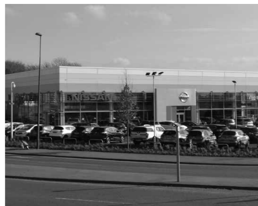
NISSAN BRISTOL CLIENT: AVIVA ROLE: Acquisition of a new to market investment VALUE: £6.03m
