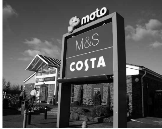
WOOLLEY EDGE MOTORWAY SERVICE AREA CLIENT: Orchard Street Investment Management ROLE: Investment valuation advice VALUE: c. £35m
