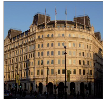
Grand Buildings, London WC2 Size: 199.230 sq ft Use: Grade A offices and retail Tenant: Enterprise Oil, National Grid and Reed Elsevier
