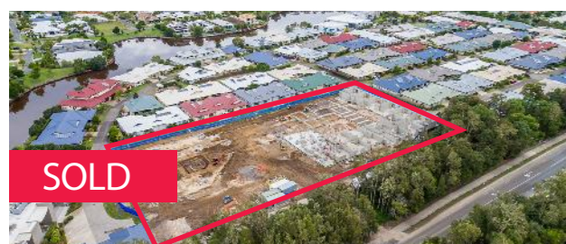
Aged Care Site Baywater Road, Twin Waters, QLD 0.94 hectare site. Aged Care site.
