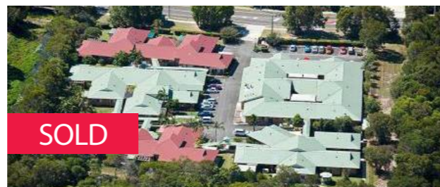
Mount Coolum Aged Care 15 Suncoast Beach Drive, Mount Coolum, QLD 120 beds Aged Care Facility.
