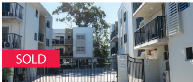
Birdwood Place Aged Care 21 Birdwood Road, Holland Park West, QLD 72 beds Aged Care Facility.
