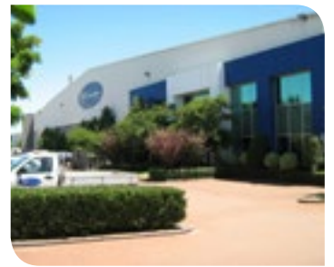
Lot 100 Pilbara Street, Welshpool
