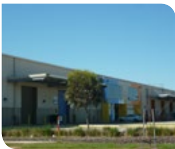
5 Butler Boulevard, Adelaide Airport
