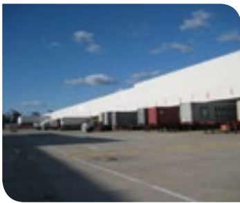
Coles Distribution Centre 2-36 Bannister Road, Canning Vale
