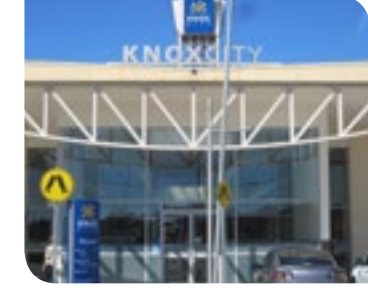
Knox City Shopping Centre 425 Burwood Highway, Wantirna South
