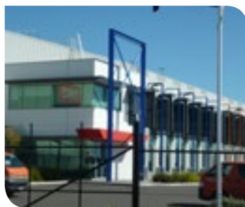
20-22 Butler Boulevard, Adelaide Airport
