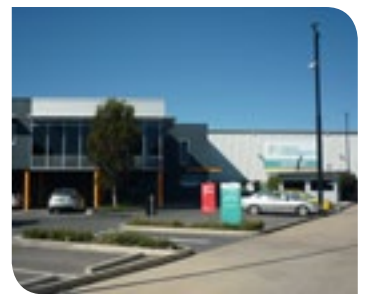
10 Butler Boulevard, Adelaide Airport
