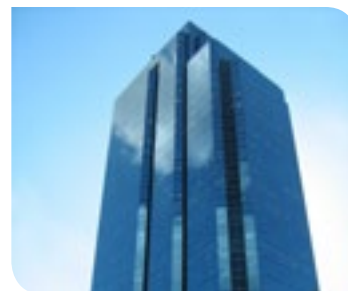
Exchange Plaza 2 The Esplanade, Perth
