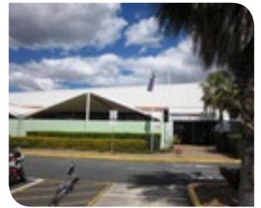
Forest Lake Distribution Centre 349 Stapylton Road, Heathwood
